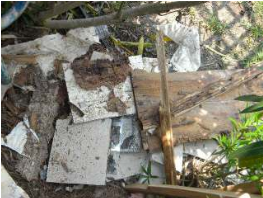
Debris pile after hard coat stucco removal
