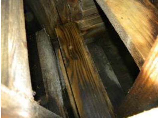
Wall cavity under a deck
