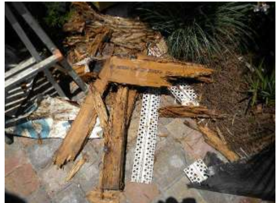
Rotted wood removal pile
